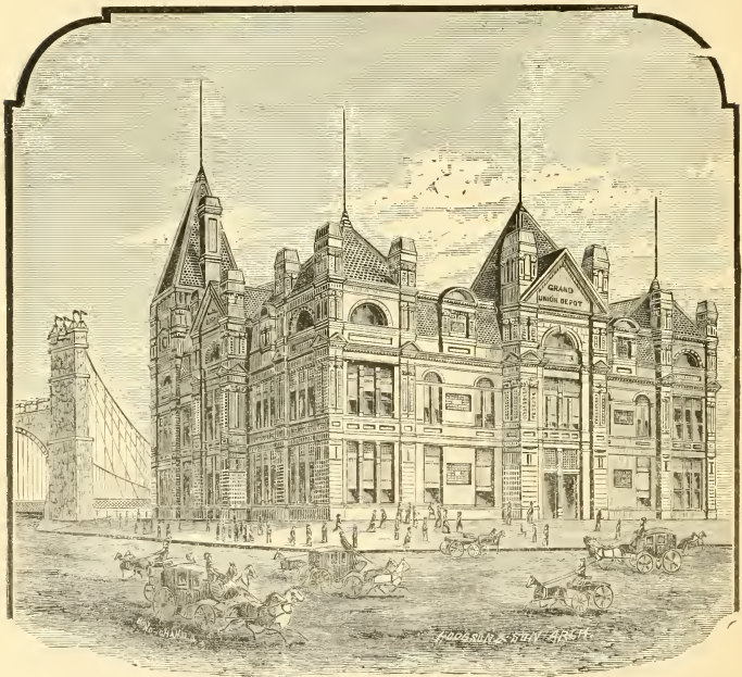
THE UNION DEPOT. (IN PROCESS OF ERECTION.)
